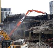
The Shopping Centre North has now been demolished and all demolition arisings stockpiled, crushed and processed for re-use on site.
